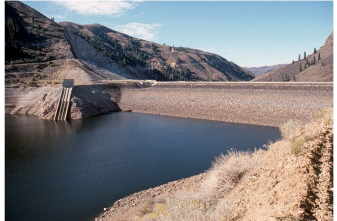
Anderson Ranch Dam and Reservoir
